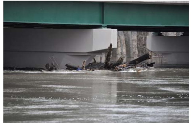
(Hwy 41 Bridge - Photo Courtesy of Jason Kirsch)
